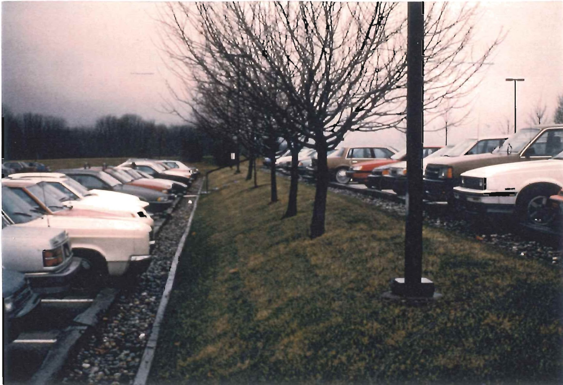
Porous paving (to left of white line) infiltrates rainfall and runoff from impervious paving (to right of line).
