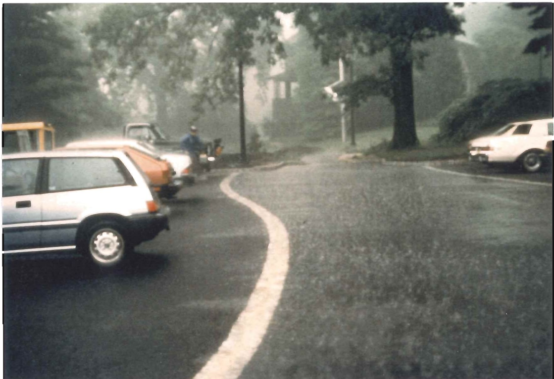
Porous paving (to left of white line) infiltrates rainfall and runoff from impervious paving (to right of line).
